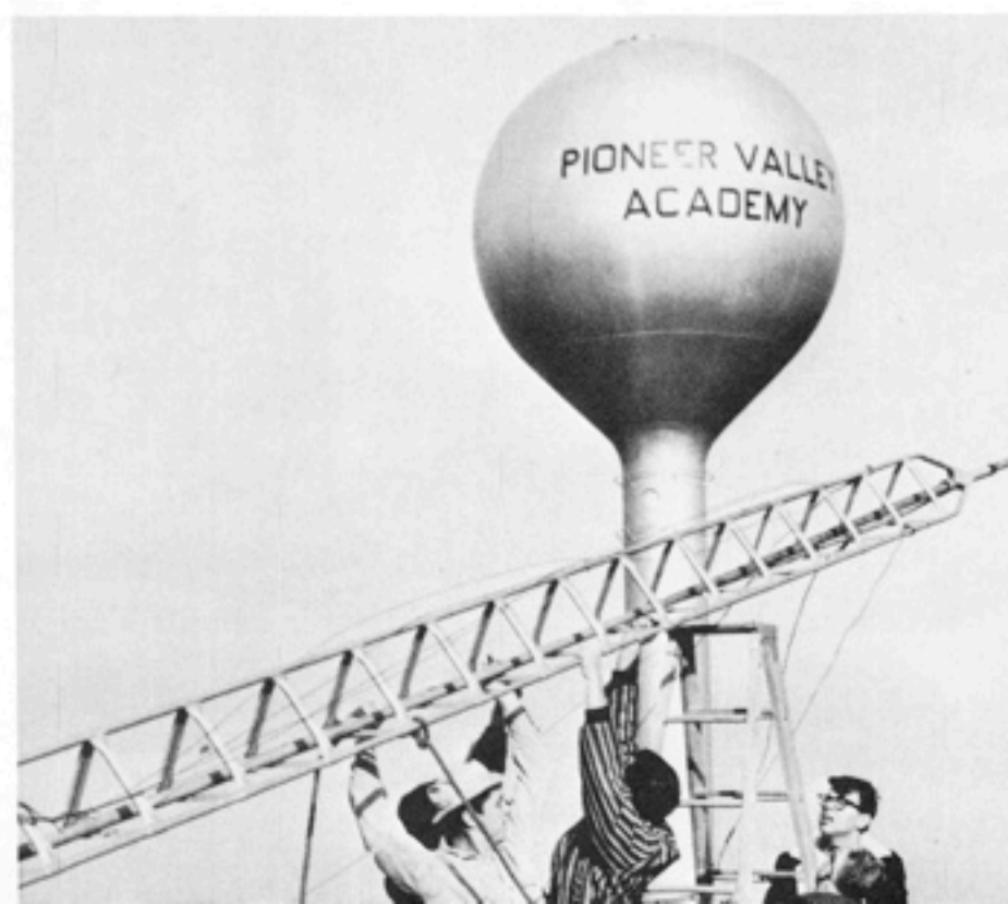
Raising the radio tower.
